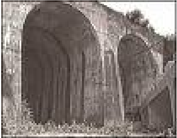
The bridge at No Gun Ri
