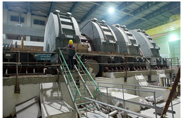
The Bushehr nuclear power plant
