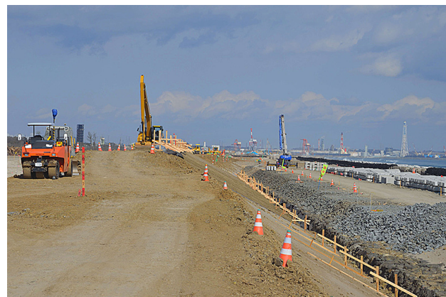
Seawall construction in Sendai, in Miyagi Prefecture, which was hard-hit by the 2011 tsunami. Conservationists and some scientists say the Japanese government could be doing far more to sustainably rebuild its coastal storm defenses, including constructing seawalls further inland, where they won't fragment marshes, dunes, tidal flats, and beaches. (Photo by Winifred Bird)
