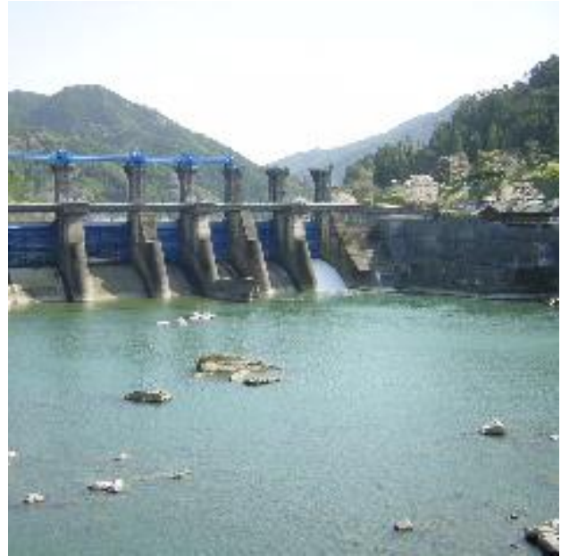
The Arase Dam
