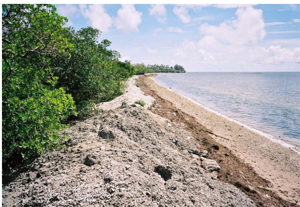
The low-lying coastline of Tongatapu, Tonga. A combination of an earth embankment and vegetation might stave off erosion in the short-term. (Image credit: Ilan Kelman)
