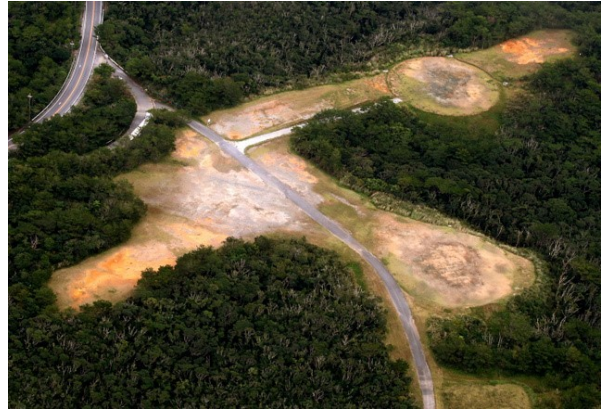
Gouged Forest and Completed “Osprey Pads”
