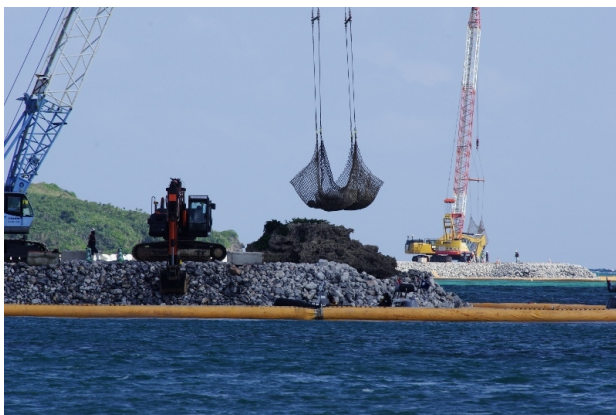
K-1 and N-5 Seawall Construction, © Yamamoto Hideo
