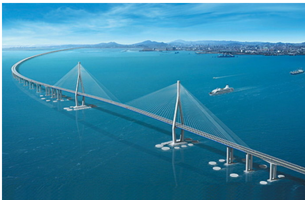
Incheon Bridge connecting Songdo to the International Airport
