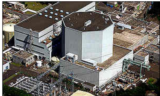
Tsuruga reactor, site of a 1999 leak
