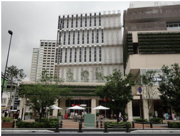
The "energy building" in Gate Square equipped with a rechargeable battery system and the power interchange unit (source: Nikkei BP)
