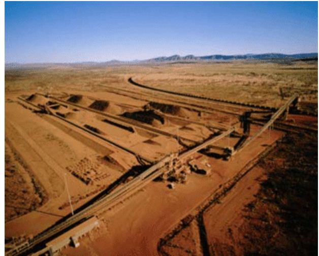
The West Angelas Mine
