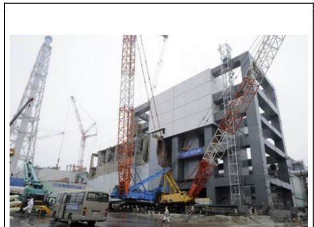
Tepeco preparing to remove irradiated fuel
