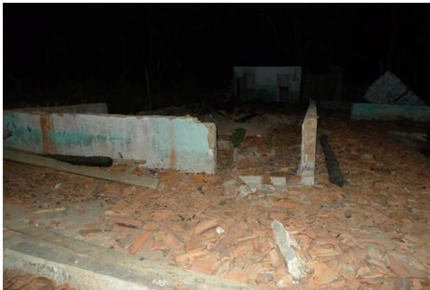
Destroyed Shi'a house at Nanggernang hamlet, Karang Gayam village, Omben, Sampang, Madura
