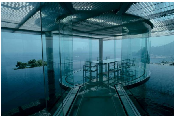
Making a connection: Kuma Kengo's 'Water/ Glass' structure in Atami, Shizuoka Prefecture, attempts to connect architecture with the sea by means of a veranda of water. | MITSUMASA FUJITSUKA
