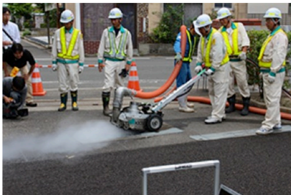
Decontamination work at Fukushima University
