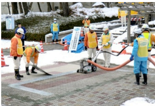
Decontamination work at Fukushima University
