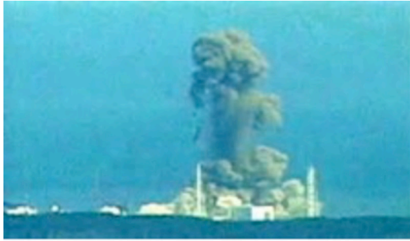
Explosion at Fukushima Daiichi Nuclear Power Plant March 2011
