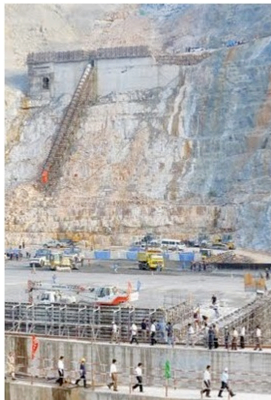
Kamchay Dam under construction
