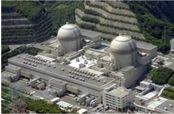
The Oi reactors may be sited on an active fault-line
