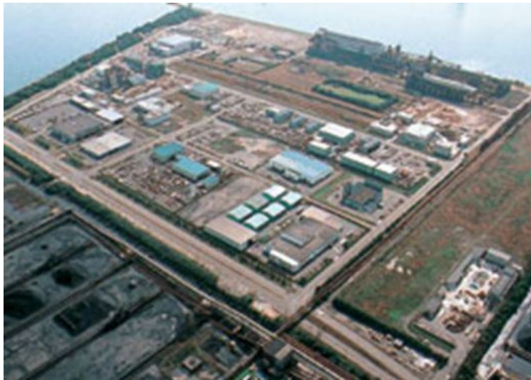
Kitakyushu's eco-town under construction
