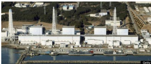
Fukushima Daiichi Nuclear Power Plant (before)
