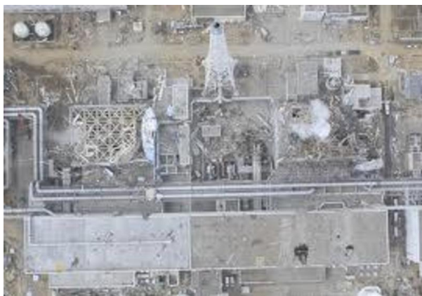
Fukushima Daiichi Nuclear Power Plant (after)
