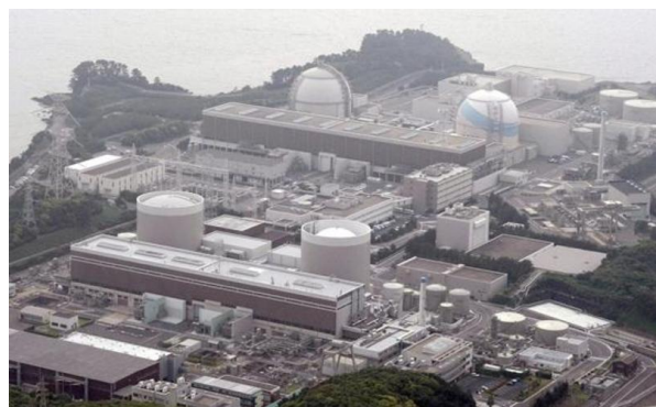
Genkai Plant's 4 Reactors are Close Together
