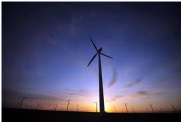
Wind turbines in Gansu
