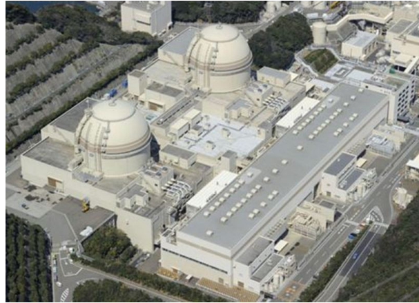
Buildings housing Oi reactors 3 and 4 in Kyodo photo in 2000
