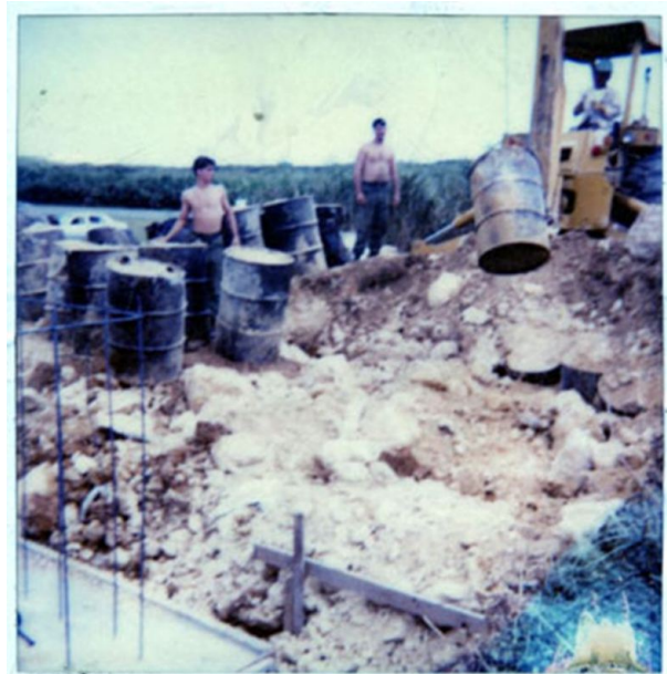
Deep deception: The worksite where Kris Roberts unearthed over 100 leaking barrels is seen in a photo taken in summer 1981. KRIS ROBERTS
