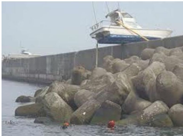
In Tohoku, seawalls and tetrapods were overwhelmed
