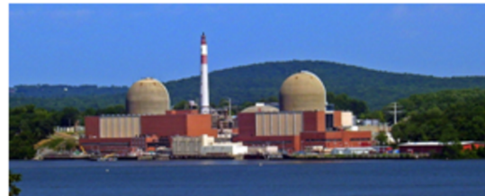
Indian Point Nuclear Power Plant
