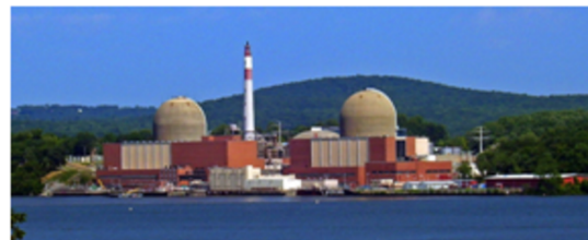
Indian Point Nuclear Power Plant
