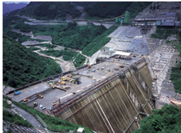
Takizawa Dam, second construction
