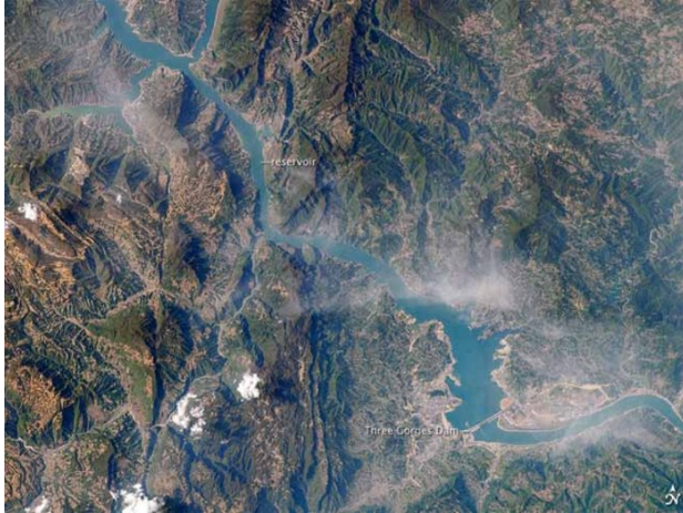
A view of the dam from the International Space Station, June 3, 2009
