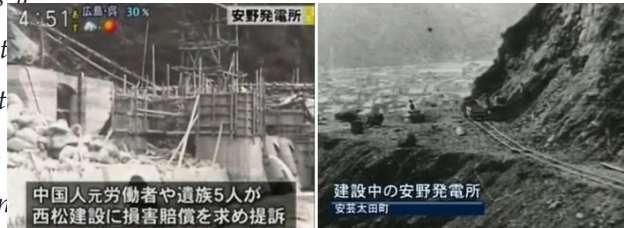
War-time images of construction site for Yasuno hydroelectric plant
