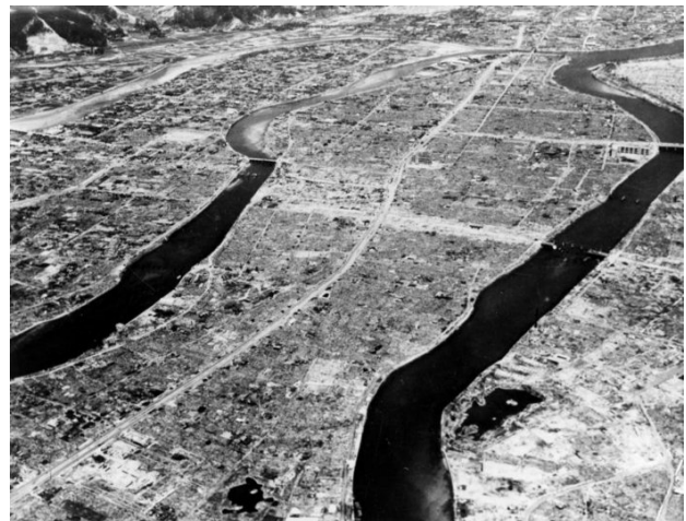
Aerial view of Hiroshima after the bombing.
