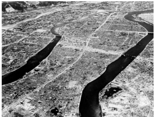
Aerial view of Hiroshima after the bombing.
