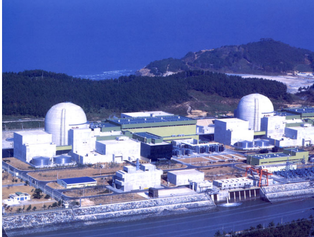
ROK Yonggwang Nuclear Power Plant
