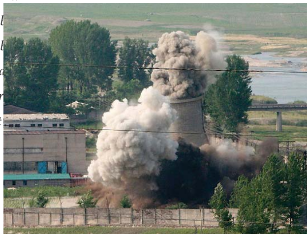
Cooling tower explodes at Yongbyon
