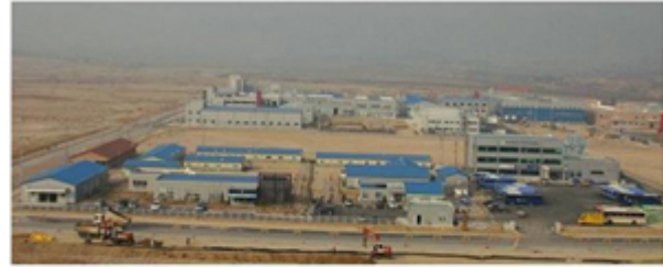
<Gaeseong Industrial Complex>
