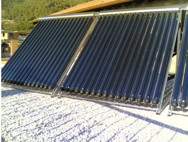
Solar thermal collector, China
