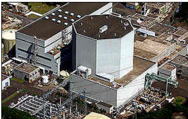
Tsuruga reactor, site of a 1999 leak
