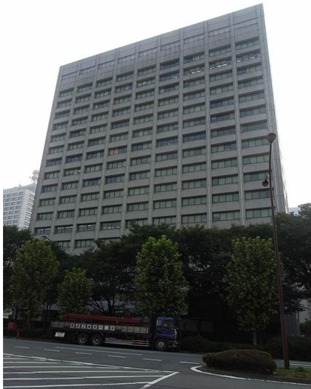
METI headquarters in Kasumigaseki
