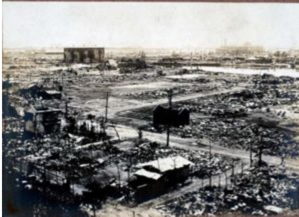
Earthquake destruction in Yokohama
