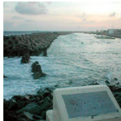
Exporting tetrapods. A tetrapod breakwater offshore at Male, capital of the Maldives. The plaque notes that Overseas Development Aid from Japan provided the tetrapods.
