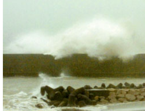
Tetrapods in action during a July typhoon that hit Kyushu.
