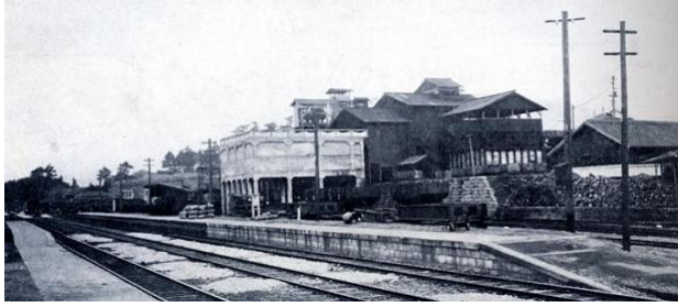
1933 photo of coal sorting equipment at Aso Yoshikuma mine in Keisen town, Fukuoka (Kyushu University Digital Archives)
