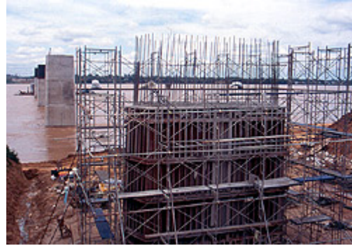
Second Mekong Friendship Bridge in construction
