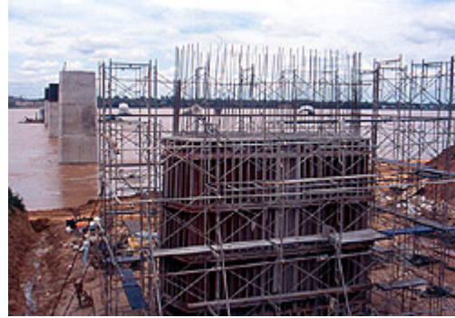
Second Mekong Friendship Bridge in construction
