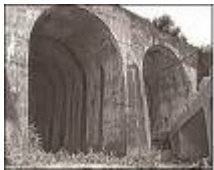
The bridge at No Gun Ri
