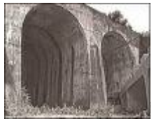
The bridge at No Gun Ri
