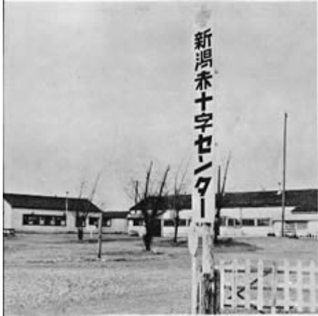
Japan Red Cross Center in Niigata
