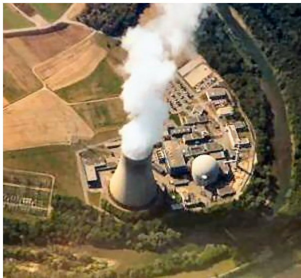
Nuclear power station at Leibstadt, Switzerland
