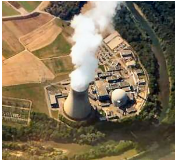
Nuclear power station at Leibstadt, Switzerland
