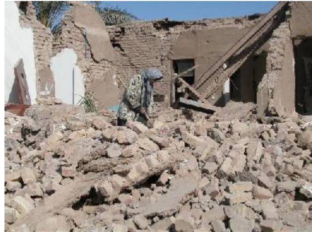
Bam Earthquake on Dec. 26, 2003.
