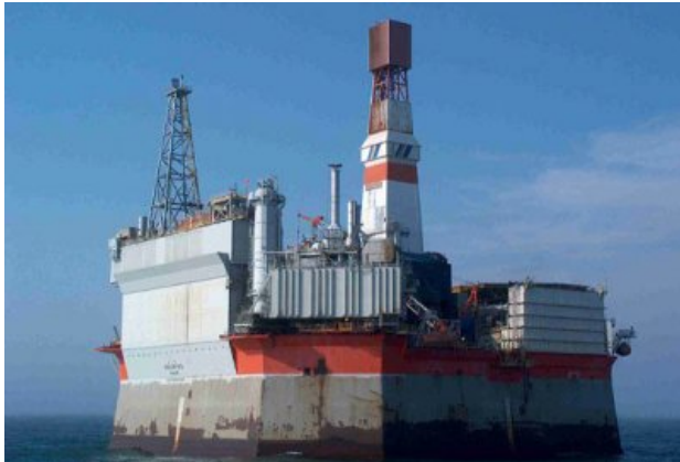
Molikpaq offshore platform currently used for producing oil at Sakhalin-2
