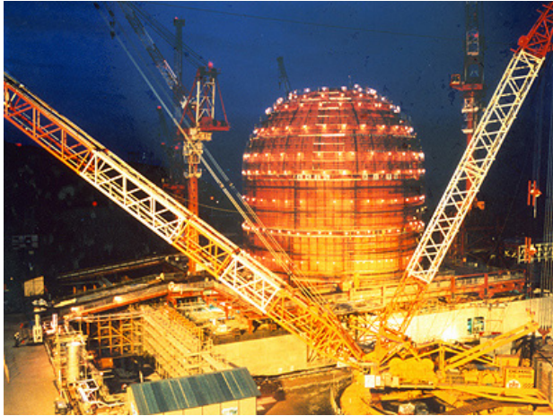
Plant under construction at Tomari
