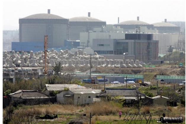
Four nuclear reactors at the Wolsong Nuclear Power Plant. Photograph by Lee Jin-man
