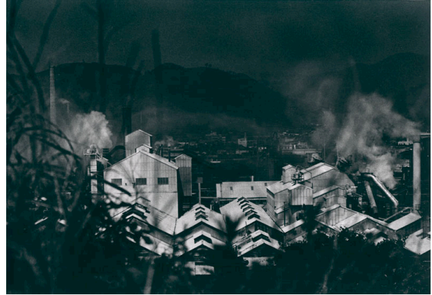
The Chisso Minamata plant
