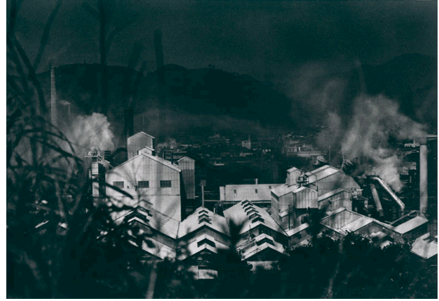
The Chisso Minamata plant
