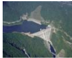
1. The Miyagase Dam
