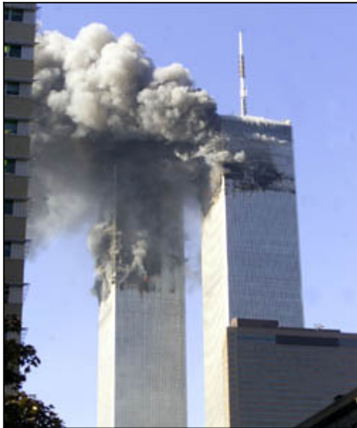
Twin Towers burn after plane attacks
