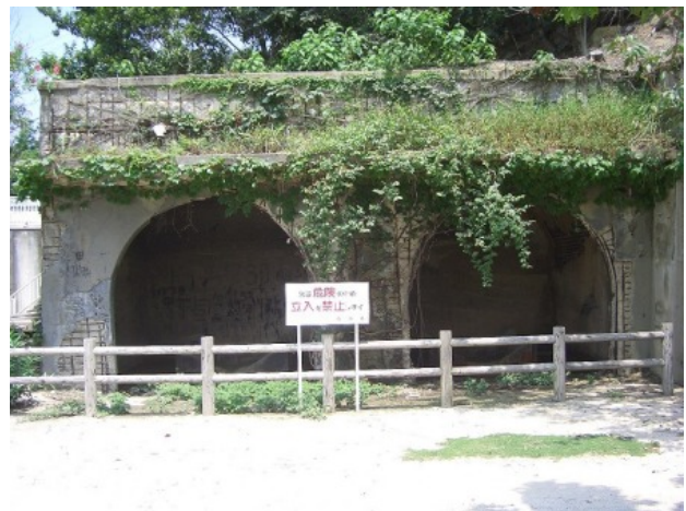
2. Storage Facilities for poison gas.
