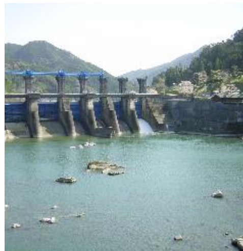
The Arase Dam
