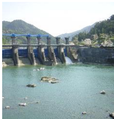
The Arase Dam
