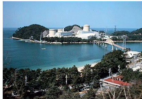
Mihama Nuclear Power Plant
