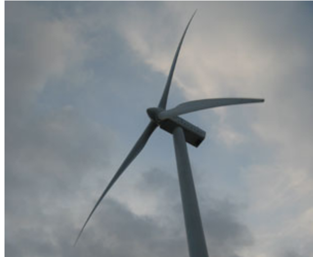
Yokohama's wind turbine
